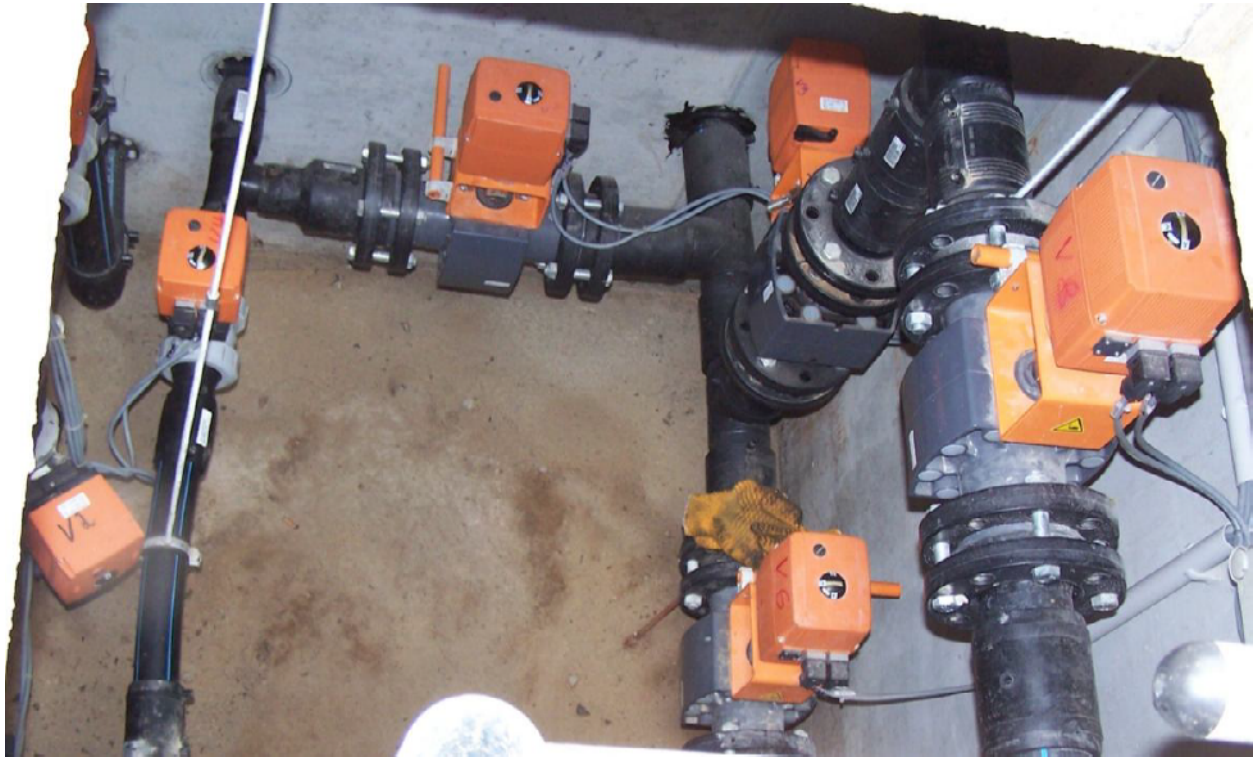
Figure 2 An additional fitting shaft ensures the redundancy of the plant components for watering
